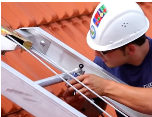
Fig. 33 Assembly upper limit switch
